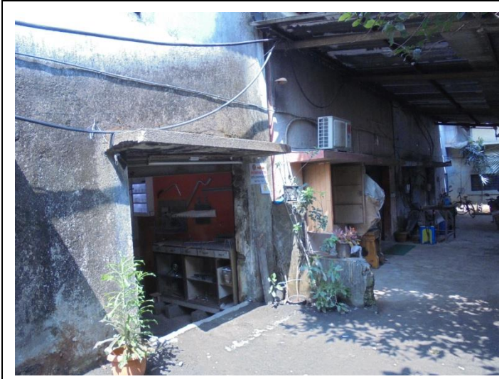
Factory Area Overview
